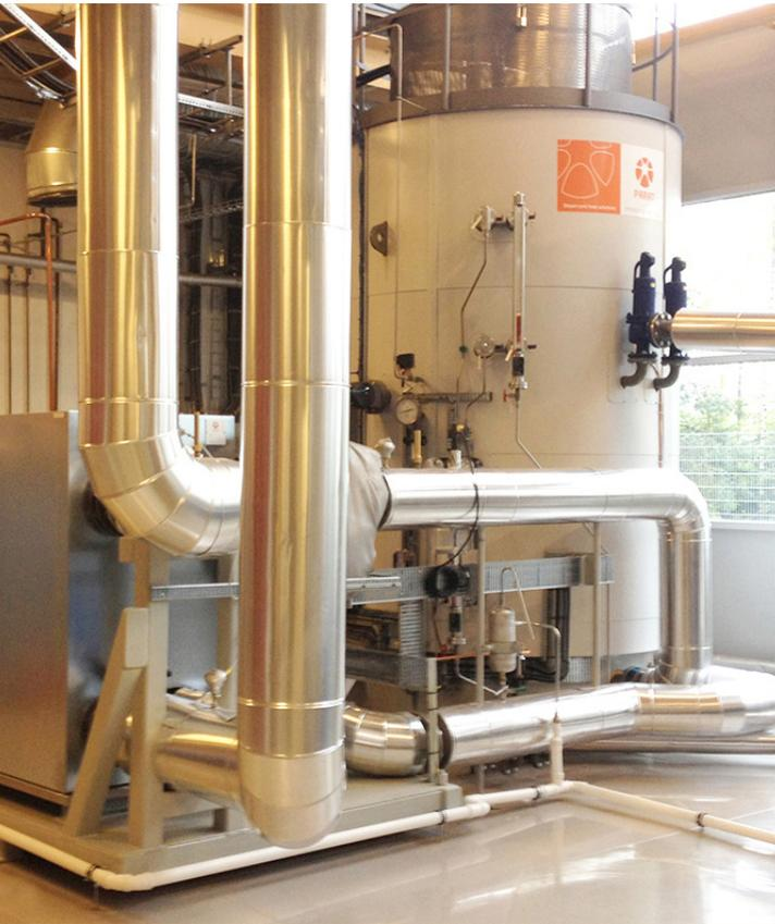
In the Ypenburg district of the Hague, houses and offices are heated with district heating. This is residual heat from electricity production and heat from gas boilers. The electricity and heat are produced with natural gas, which releases CO<sub>2</sub>. Because Eneco wants to reduce CO<sub>2</sub> emissions, from now on some of the heat will be produced with the e-boiler.
