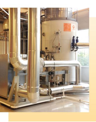
In the Ypenburg district of the Hague, houses and offices are heated with district heating. This is residual heat from electricity production and heat from gas boilers. The electricity and heat are produced with natural gas, which releases  $\mathrm{CO}_2$ . Because Eneco wants to reduce  $\mathrm{CO}_2$  emissions, from now on some of the heat will be produced with the e-boiler.
