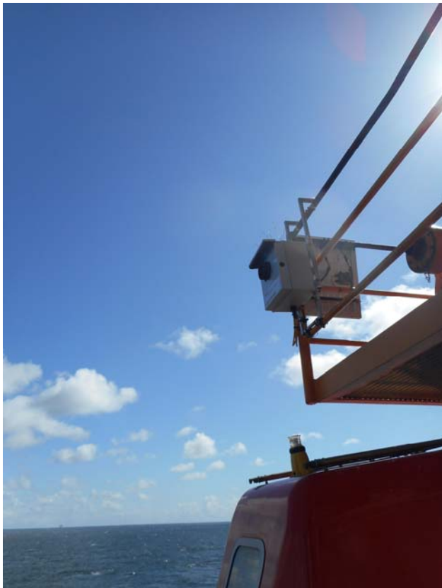
Figure Annex 1-14. Monitoring location K12-BP Platform (photo: Engie E&P)
